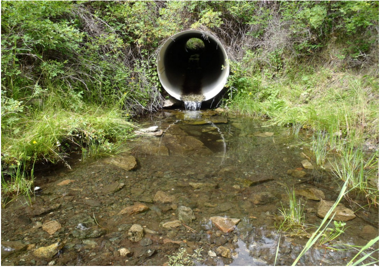
Blue Cr upper culvert outlet
