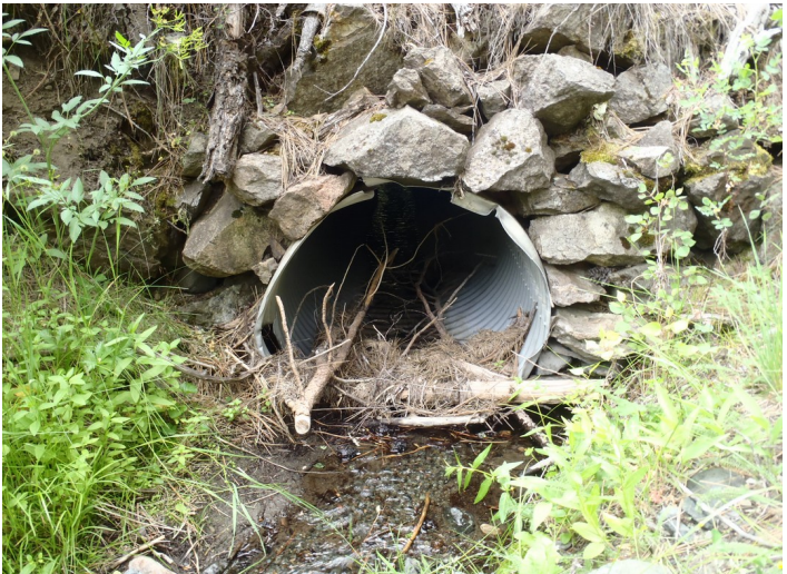
Blue Cr upper culvert inlet
