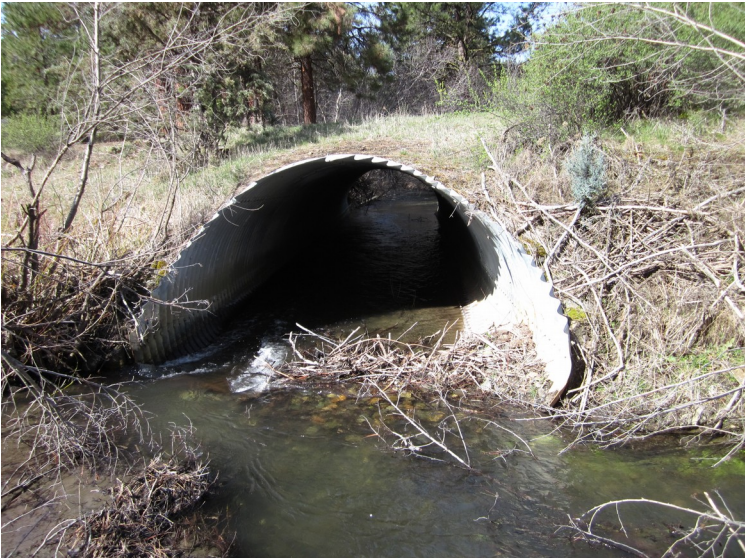
Inlet can become blocked by debris and beaver dams
