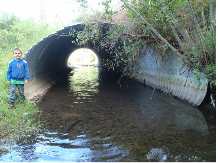
Deer Cr culvert at Buck Cr Road outlet- PASSABLE
