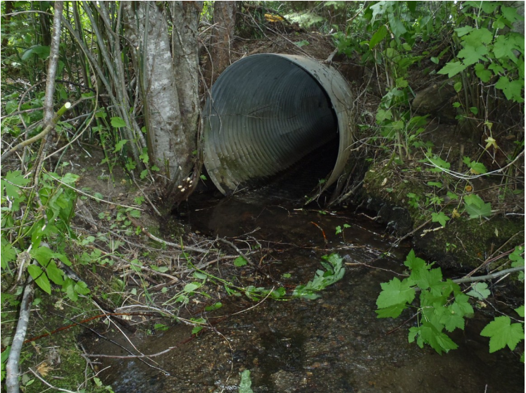
Intlet showing misalignment with stream
