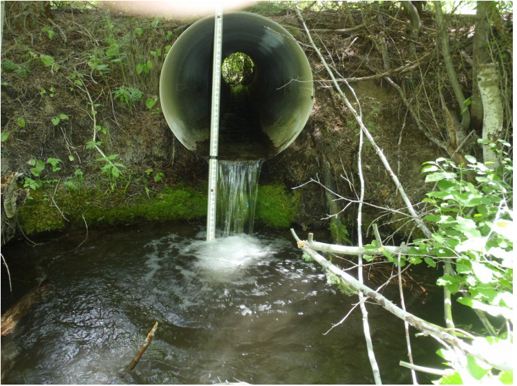
Sugar Cr culvert outlet
