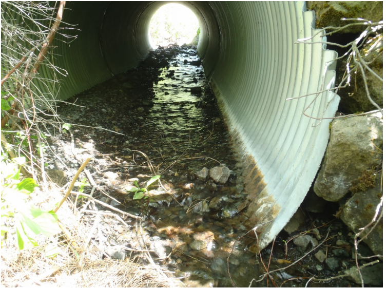
Culvert outlet showing no perch and stream bed material through its entire length
