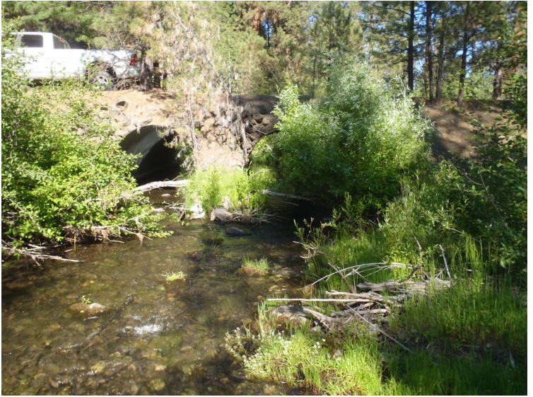
Culvert inlet showing no passage problems
