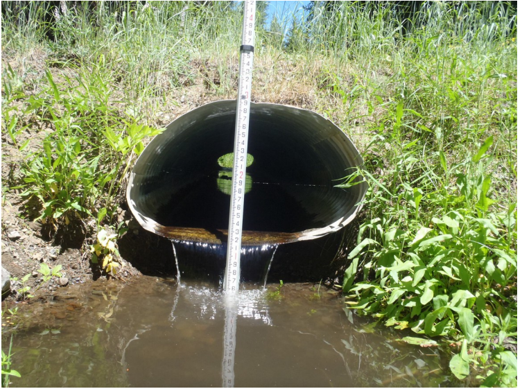
Culvert outlet showing flat slope and gravel substrate inside of culvert
