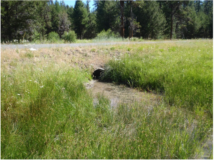
Culvert inlet and road surface
