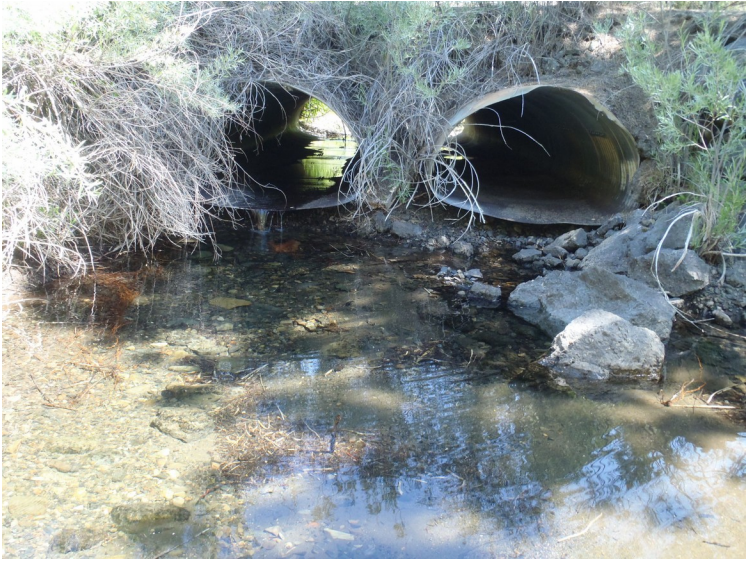
Outlet of culverts showing stream bed substrate through their entire length
