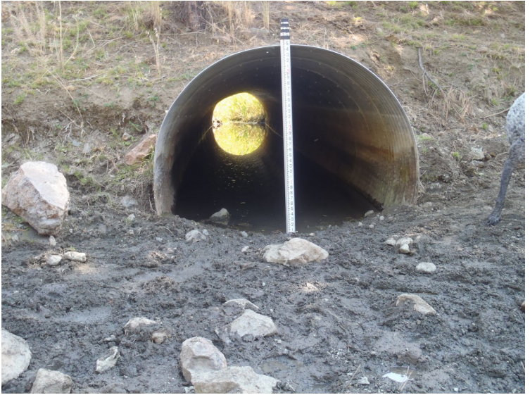
Culvert outlet is dry here but stream bed material covers the bottom
